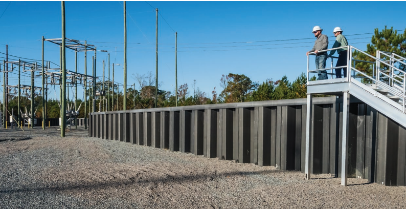
Permanent flood barriers at Duke Energy's Nichols 115-KV substation in South Carolina
